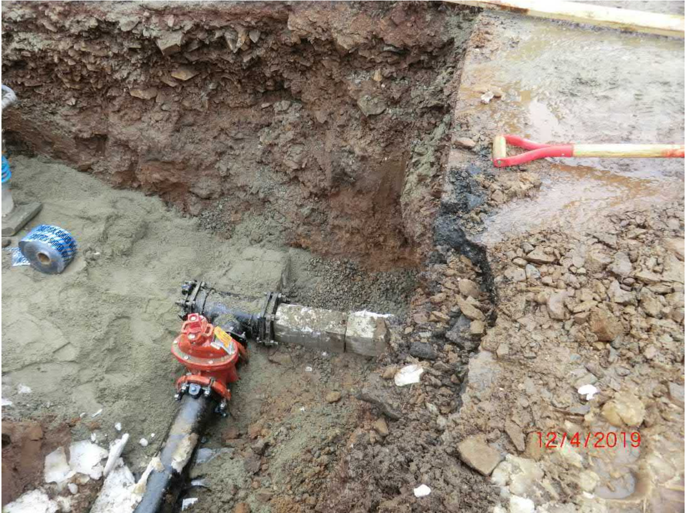
Figure 15 – Facing south into trench. End of lateral thrust blocking. Red 6” gate valve leads to hydrant, off bottom of picture.
