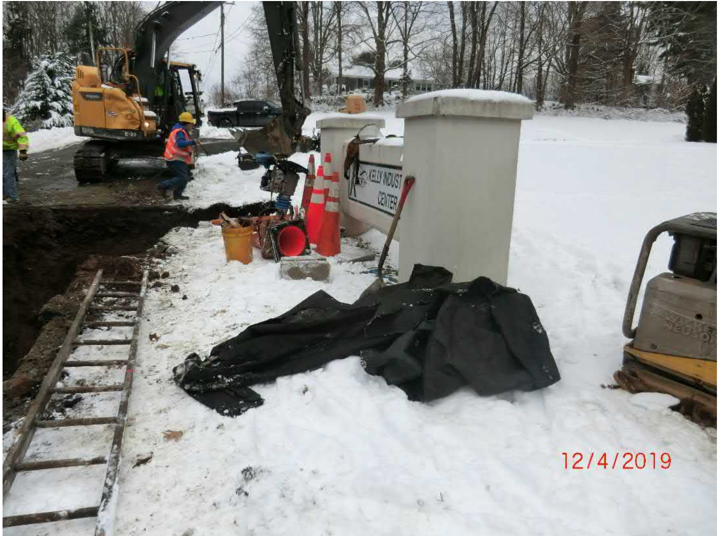
Figure 8 – Facing west up Parsons St. Turn for new hydrant. Hydrant will be set just beyond the business sign in center of shot.
