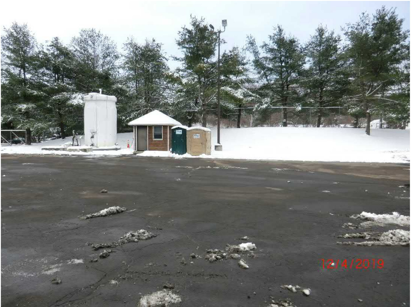
Figure 6 – Facing east northeast. CT DOT yard cleared of equipment and materials. Appears that all materials and equipment have been moved down to the MMC site (trailer area).
