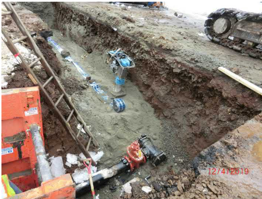
Figure 13 – End of 24 feet of 8” restrained DI pipe. End is 8x8x6 Tee with gate valve installed to feed hydrant installation to right of top picture.
