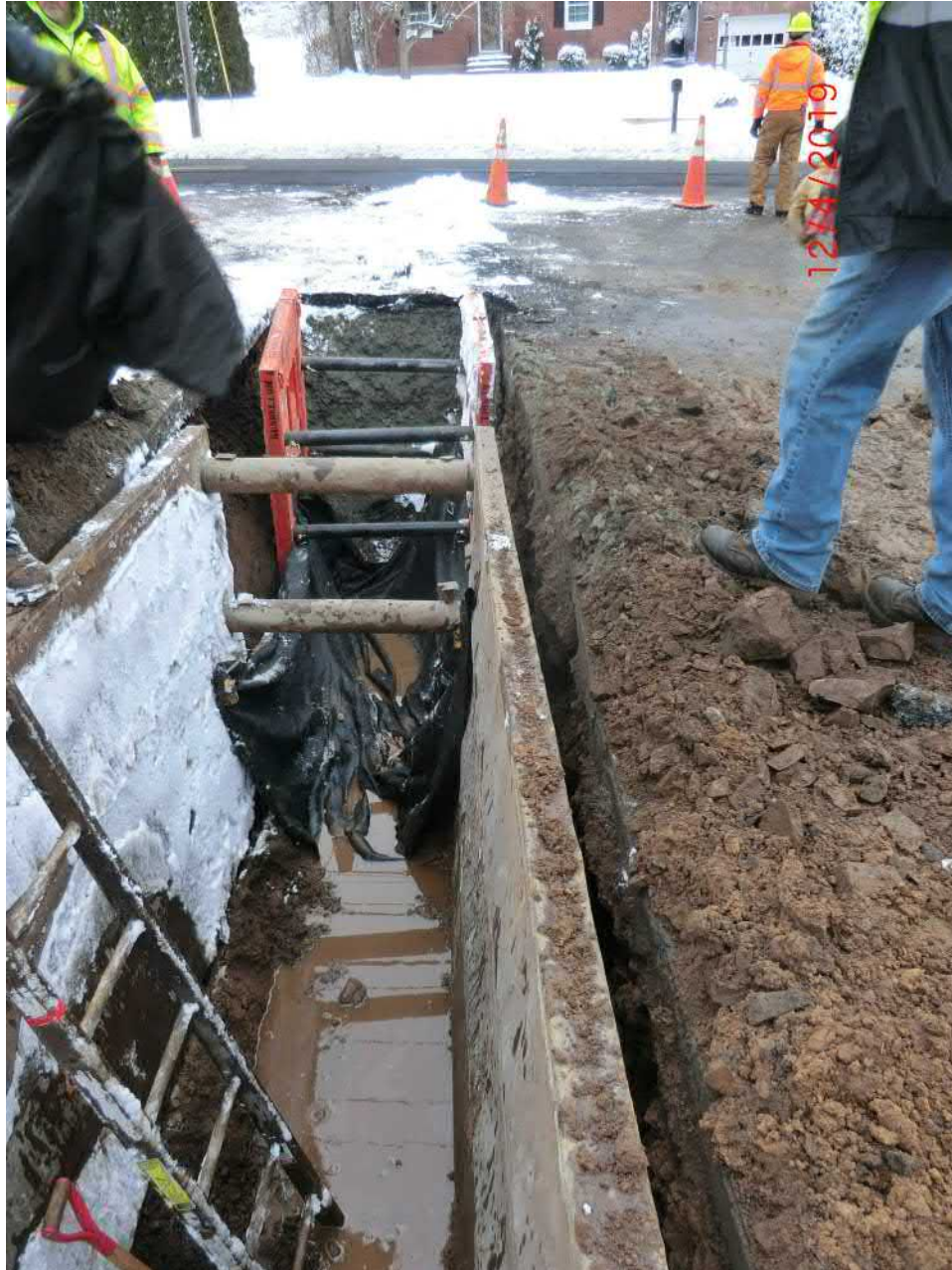
Figure 7 – Facing east. Bringing 6” DIP to hydrant. Note that the starting point is out of the State ROW. A section of pipe was added last week to get the hook-up out of the ROW for hydrant install this week. Pipe in trench is just above the groundwater line. Picture shows the installation of the stone ‘burrito’ that will underlay the 6” DIP.
