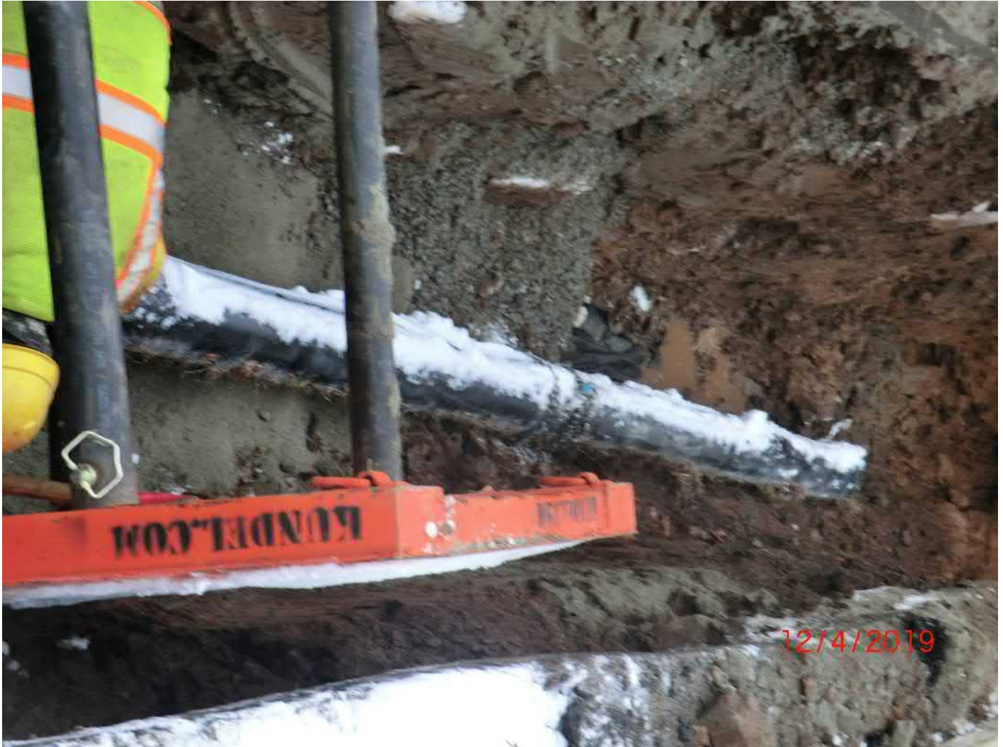
Figure 9 – Installing 20 feet of 8” DI pipe with restrained fittings.
