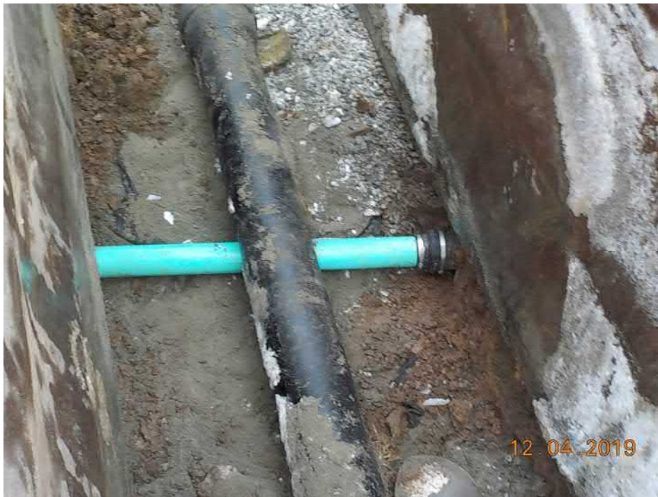
Figure 12 – Drain line repair: 4-inch PVC and Fernco couplings.
