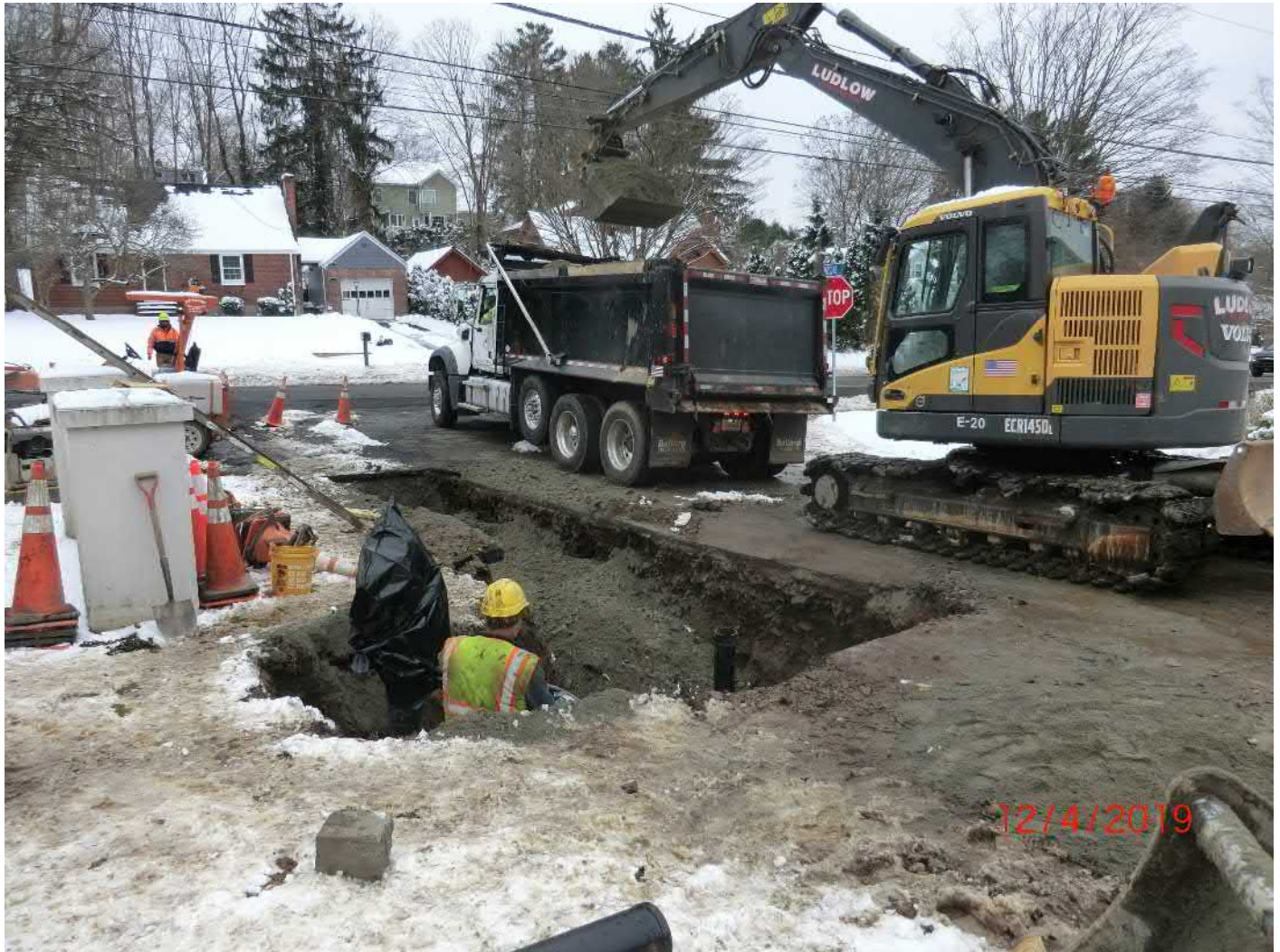
Figure 17 – Entire installation trench. On far end is connection to lateral (off Main St. line) previously installed last week to bring connection point outside of State ROW for Route 17 (Main St.). On near side is hydrant (covered in plastic). In center of picture (roughly) is the valve box. On bottom right corner of picture just above the date stamp is the sand that was laid down on the small gas spill. The sand is to be removed later.
