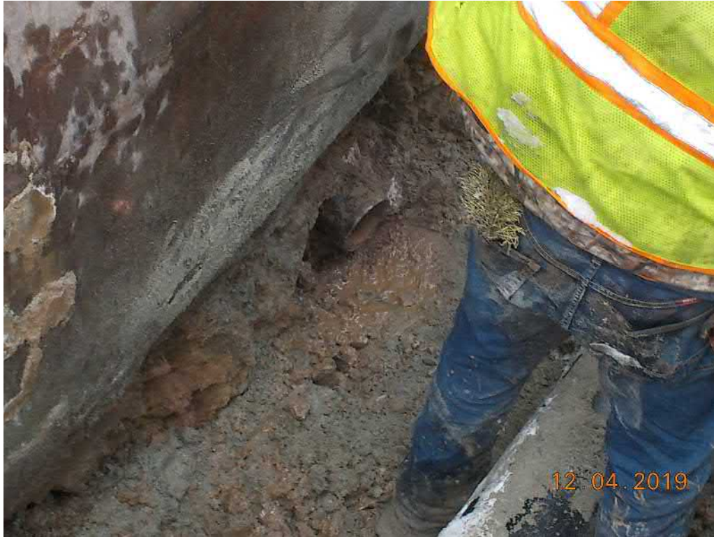
Figure 11 – Unexpected 4-inch drain line cutting across Parsons St. Cut out during excavation for lateral line off of Main St.
