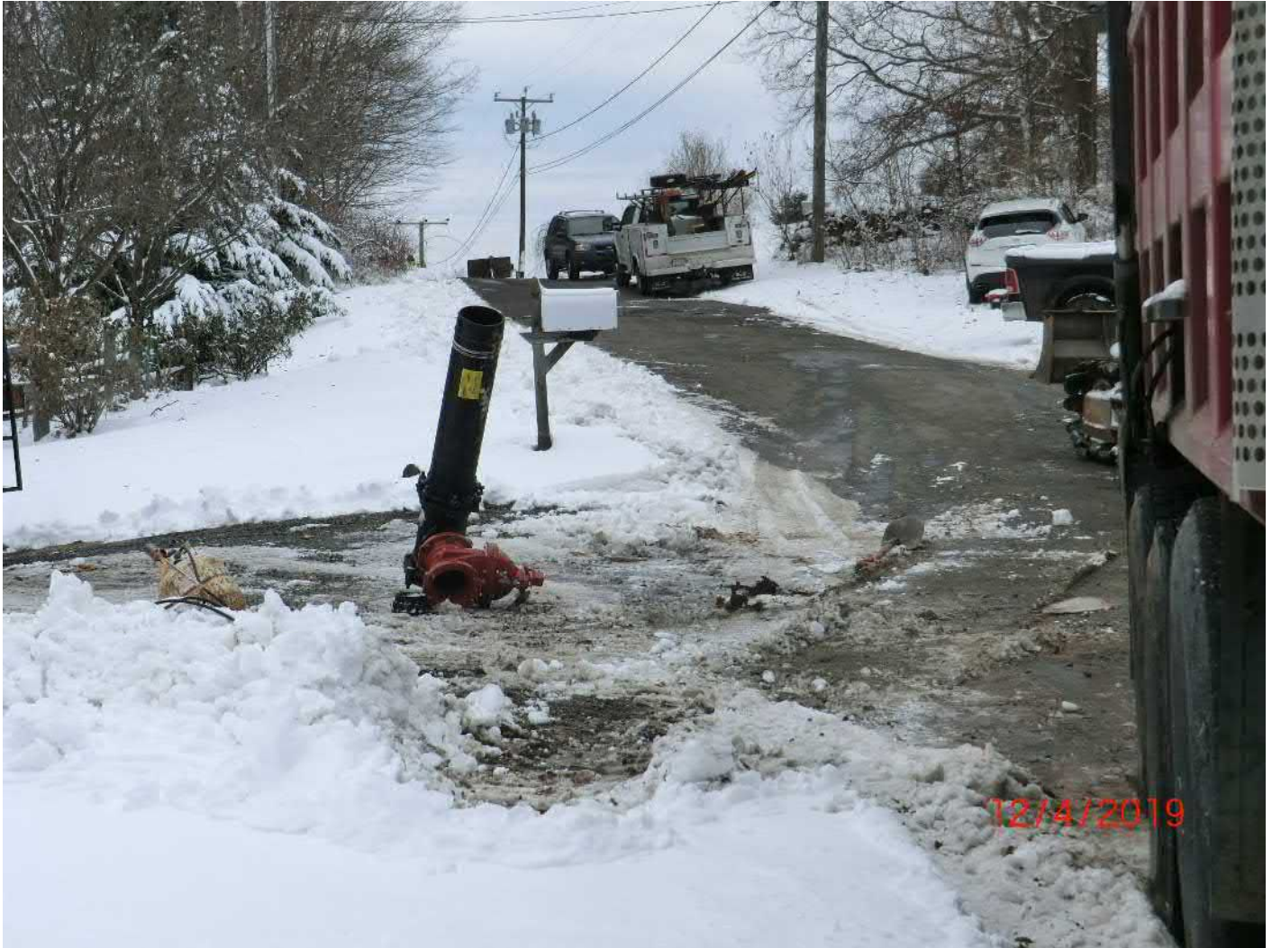
Figure 10 – Facing west. Additional 4.5 feet of 8” DIP, 6” gate valve, and 8”x6” Tee to be installed to end of stick seen in previous figure.
