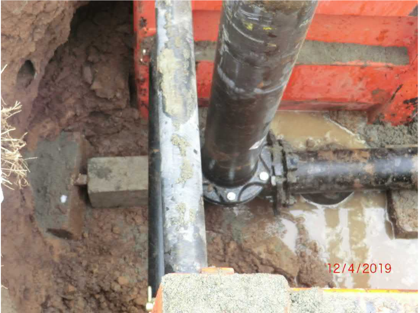
Figure 16 – Thrust blocking behind hydrant elbow. Also note support blocking for hydrant lateral on right side of picture. Shimmed blocking under hydrant elbow is not visible in this picture.
