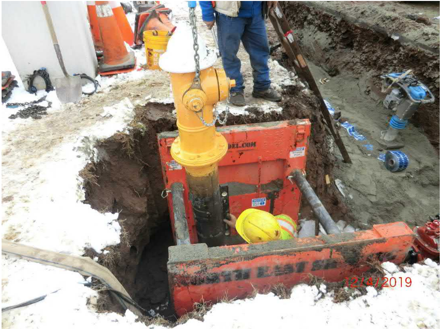
Figure 14 – Setting hydrant and checking for plumb.
